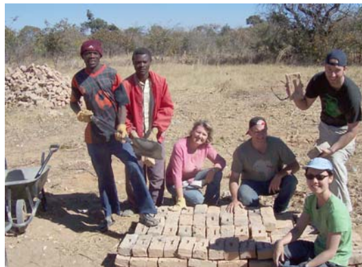
Everyone helped sort and stack the bricks - it was a team effort
