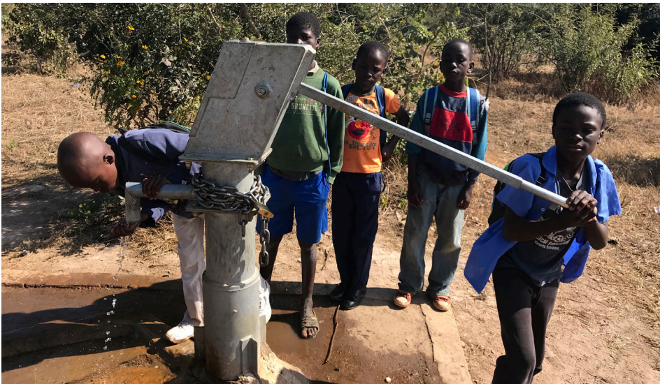
Our previous bore hole (well) was only 30 meters deep and often dried up. Our new bore hole and hand pump are drilled down 50 meters, which means we will get water even during the dry season. We plan to connect a water pump to the new phase 3 electrical connection so we can water our garden and harvest fresh vegetables for our feeding program.
